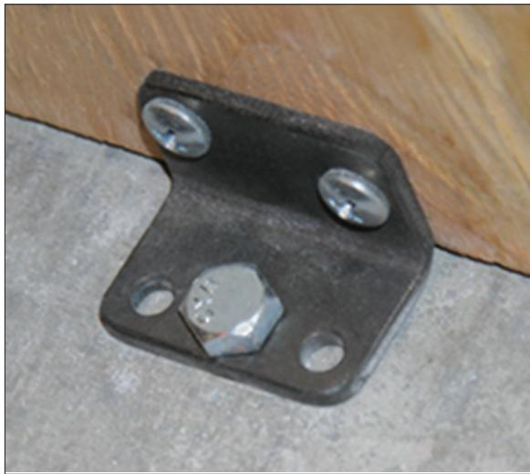
**Fig. 1** The shutter is firmly attached to a concrete floor with a Bottom Brace using a 1/4"/6.4mm lag screw into an expansion anchor. The brace can be stored attached to the shutter and the lag screw closes the anchor hole in the floor when not in use. Also works for wood floors using panhead machine screws.
